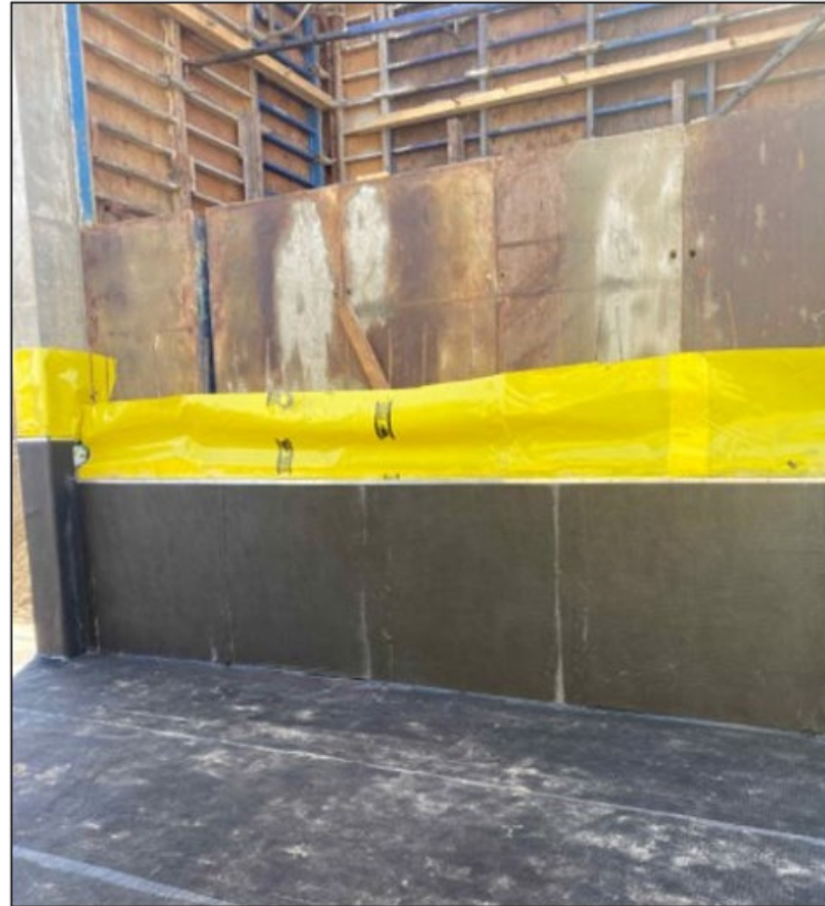
Below grade waterproofing – Site observation
