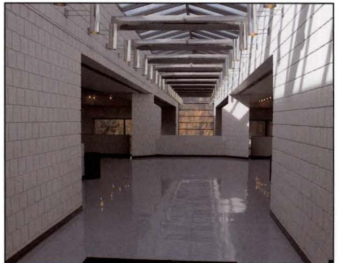
Hulbert Hall Entry Corridor
