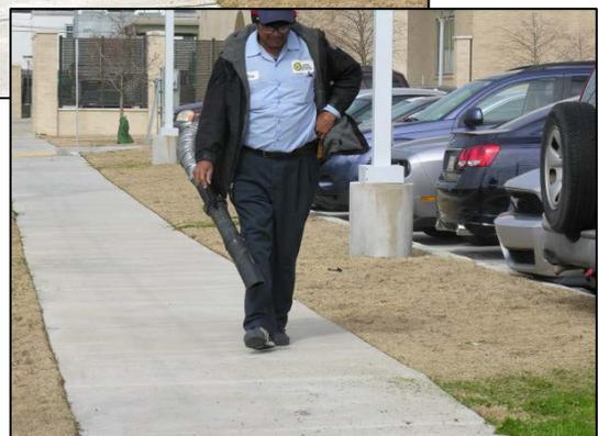
*The employee commitment to the solar PV panel and pervious pavement lots include routine maintenance such as litter removal and landscape maintenance to prevent clogged pores and decreased stormwater runoff.*
